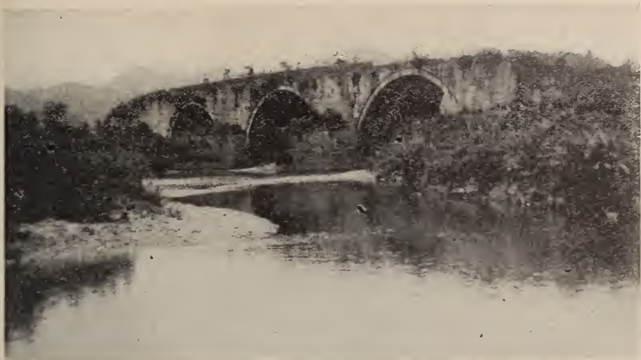
AN OLD BRIDGE
